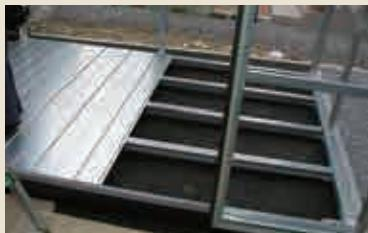
▶根太床、床板施工。□-60×60の根太床に
